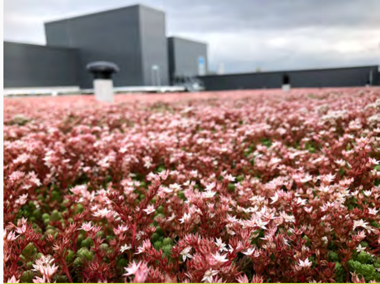
Completed Sedum Roof installed to mission critical facility, Dublin, Ireland
